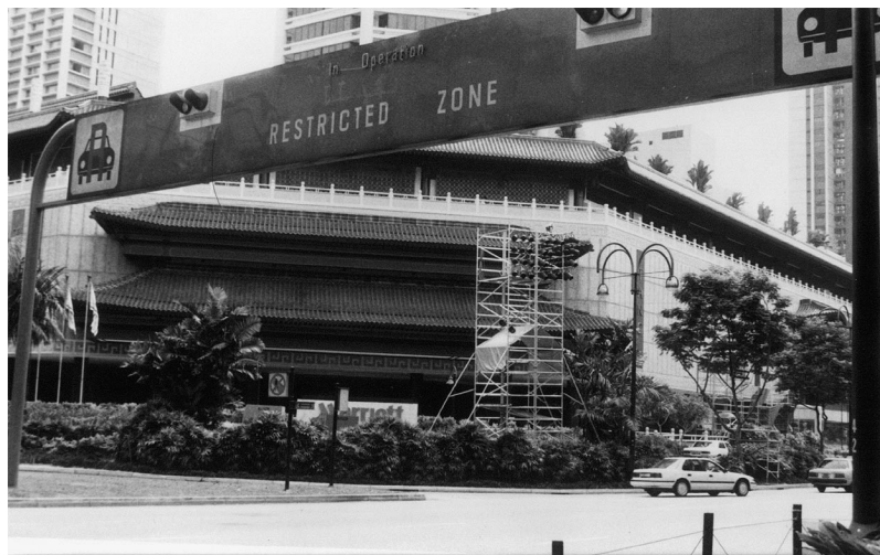
Figure 1 View of an overhead gantry used in the Area Licensing Scheme
