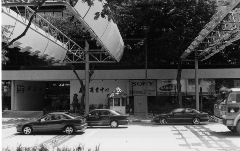
Figure 4 A side view of the pair of overhead gantries
